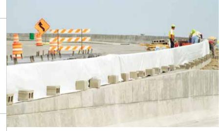
Conkure Wet Curing Blanket from Strongman consists of a highly absorbent synthetic needle-punched fabric coated with a white reflective film. Unlike burlap, it will not rot or mildew.
